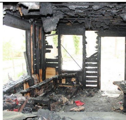
Figure 11 – Rear door exit inside dining room.
